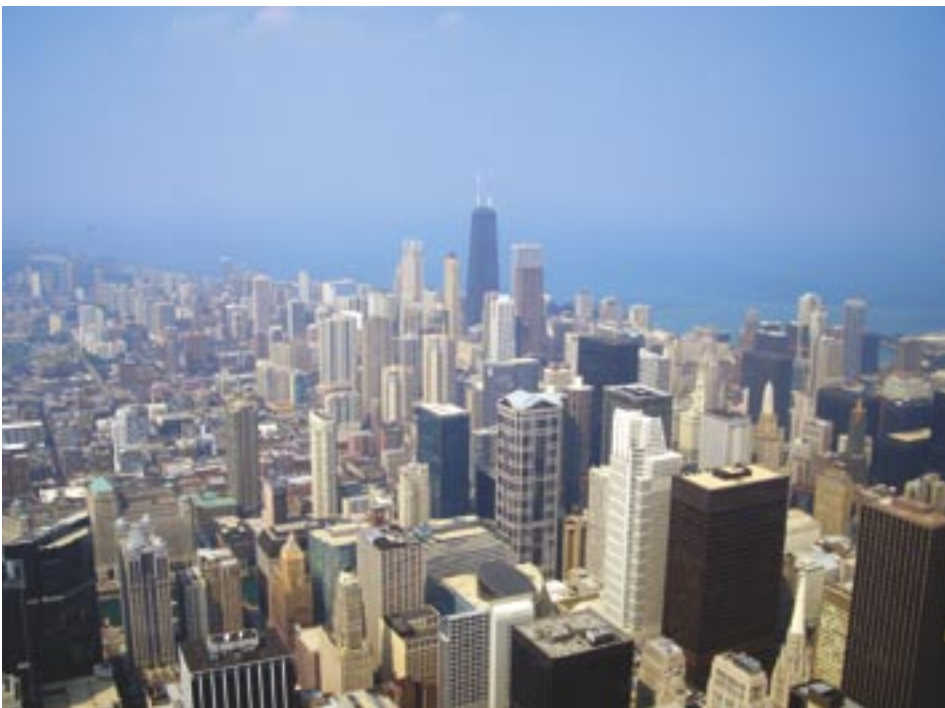
The first building erected after Chicago was razed by the great fire of 1880 was a realtor's office the size of a street kiosk marked only with a big, bold, plot-number. What has changed? Chicago had a Beaux Arts plan by Daniel Burnham. It was the ontological mauvais foi of 'functionalist'- aesthetics which allowed the CBD to fall into the hands of illiterate realtors.
