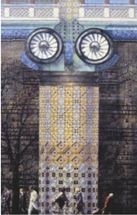
The 'Owl' capitals for Blackfriars. As 'solar wheels', they made the mechanicals of ventilation subservient to the iconology of 'flying' and 'moving'.
