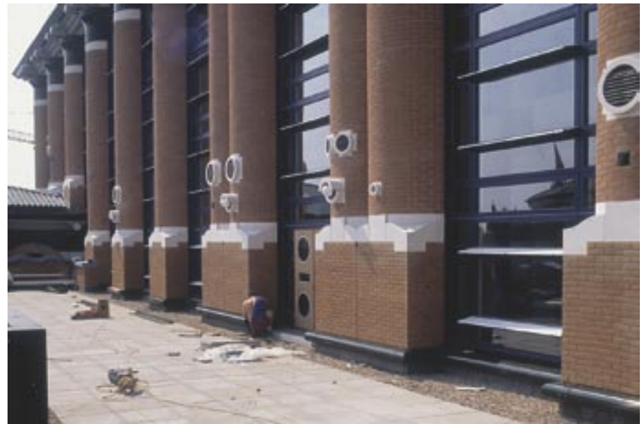
Sundry orifices in the columns along the Ark Roof Garden in the Judge Institute. These seek no 'other' identity than to manifest the 'hidden Robotism'. All are 'ruptures' to the enclosing brick skin which are necessary to the many machines inside these Serving/Robot Columns. But the holes are disciplined' to the primacy of the Column by being 'trimmed' in black and white frames which are made to bond exactly to the Order's brick skin.
